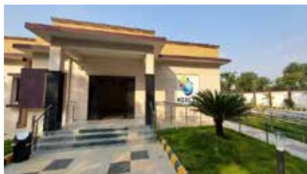
NIELIT Extension Centre, Muzaffarpur main building
